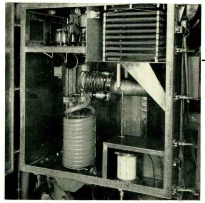
Oscillator tube with cooling system consisting of water coils and air blowers housed in movable compartment to facilitate servicing
