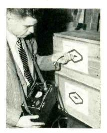
Method of using portable indicator to check condition of dessicant inside sealed package in crate
