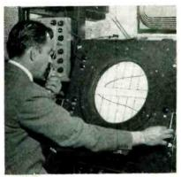
Scope presentation of airfield approaches gives ground operator plane position information from which he can direct pilot by radio
