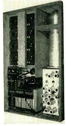
Complete gondola with radiation detector. High-voltage supply is located behind detector unit
