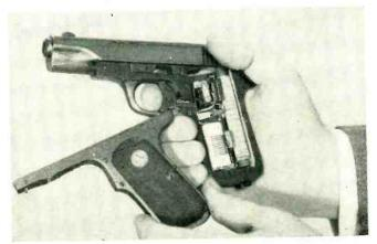
Transistor gun, showing snap-switch, transistor and battery together with inductor and capacitor in handle
