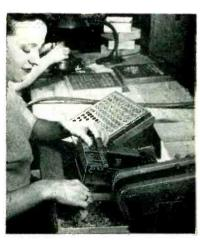
Wire-cutting setup, located at output of conveyor coming from stem machine. Bending machine is on same bench, in background
