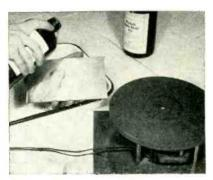
Pouring photo resist solution on copperclad phenolic sheet
