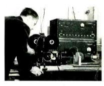
Television recording system designed for military operation comprises special film camera focused on kinescope. Ancillary electronic equipment enclosed in relay-rack cabinet is not shown
