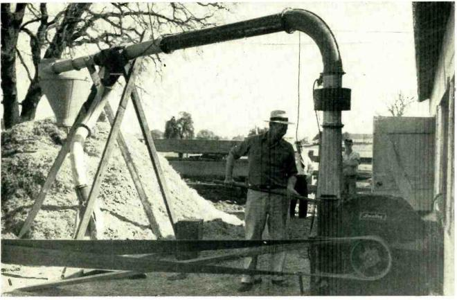
First field trial of tramp-iron remover. Total of 34 pieces of dangerous wire and nails was removed from this haystack in first pass through setup, and none on second pass
