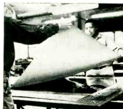
Laying sheet of pre-coated electrolytic sheet copper on polished platen of press
