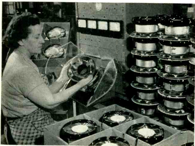
DEFLECTION yokes for color tubes roll off RCA's production line as . . .
