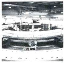
Brookhaven Cosmotron's 2432 magnet grid bars, operating in high vacuum, are "gapped" and insulated with "Kel-F" plastic.
