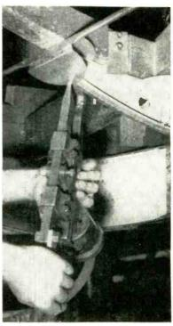
Using electric hand welding machine for welding preshaped tubing to stainless steel joint flanges which in turn are shot-welded to the vertical ribs of the radar screen. Welder is supported from ceiling on track carriage. Assembly is done on shaped wood forms having positioned brackets
