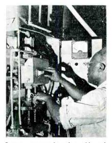
Operator removes heated crucible with tongs after power has been shut off by 30-sec timer in control box of furnace
