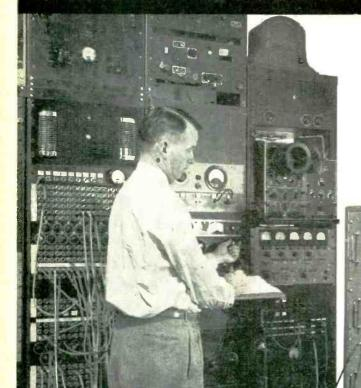
Rapid, accurate determination of transmitter and oscillator frequencies at multiple-transmitter overseas communication center.
