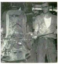
Use of three special shaping rolls to give required parabolic shape to shorter lengths of half-inch tubing. Several passes are used, with the degree of arc increased for each pass. No mandrel is needed to prevent deformation
