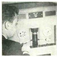
Microfilmed documents previously marked are read of by flying-spot scanner in new technique developed for computer input
