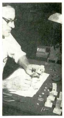
Applying No. 718 flat brazing wire to joint area during assembly of flange to a waveguide prior to dip brazing
