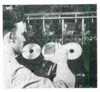
Inserting screen-faced cathode-ray tube into memory frame of computer capable of storing 1,024 twelve-digit numbers
