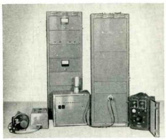
Microsecond flash equipment with high-speed camera at left. Pulse generator supplies triggering pulses for series of ten flashes
