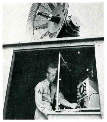
Signal Corps installation showing van-mounted radar set with antenna on roof to permit a relatively short run of output line, but even this may be too long at higher microwave frequencies. To avoid frequency-jumping, X-band output line lengths must be less than 12 feet, and K-band lengths under 4 feet
