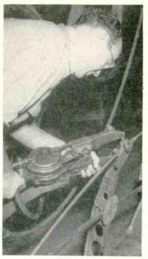
Final joining of half-inch tube members to the radar screen frame is accomplished by shot-welding the tacked joints. Lower assembly of the screen skeleton has been removed from wood shaping form and is now ready to be joined to upper assembly
