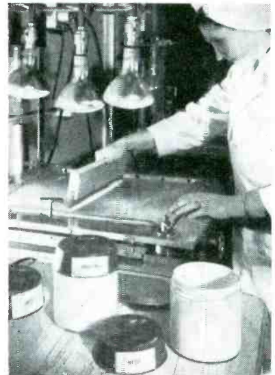
Applying blue phosphor mix to screen through gelatin stencil or frame
