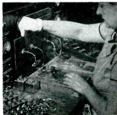
Placing solder preform over metalized bathtub capacitor loaded on slide
