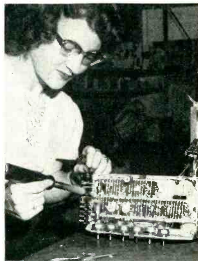
Leads are soldered conventionally to ceramic terminal strips
