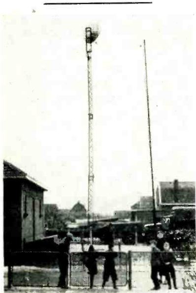
RADIO relay supplemented damaged telephone cables, as . . .
