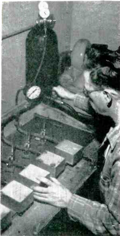
Arrangement of vacuum and gas lines for filling transformers with nitrogen
