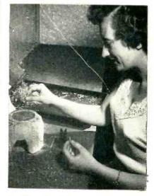
Pigtail is dipped through solder pot with a sweeping motion to minimize pickup of dross on surface. Body of capacitor is in left hand, ready for quick application to lead
