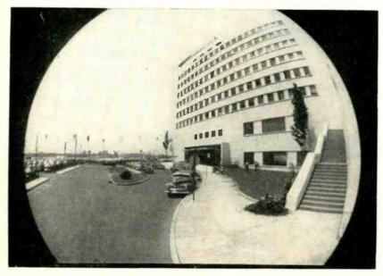
Wide-angle lens giving 142-degree field of view, as used at the Navy's Special Devices Center, Sands Point, N. Y. in a gunnery trainer. A televisian system using this wide-angle lens and a spherical-screen projection receiver to pravide three-dimensional television is presently under development at RCA
