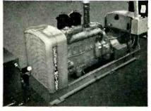
WKTV---UTICA, N. Y., uses a 100 kw. General Motors Diesel generator set far stand-by power. Set can be started remotely from the control room. Low vibration characteristic of engine permitted installation in room adjacent to transmitter and within 30 feet of studio.
