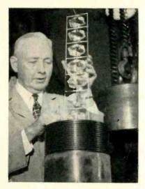
Batch of 11 perfect 160-gram quartz crystals being unloaded by A. C. Walker after growing 48 days in 4-foot autoclave at Bell Telephone Labs in Murray Hill, N. J. Threaded cap is removed with huge wrench and chain hoist, after which welded-steel inner liner is sawed open. Project is sponsored by Signal Corps Engineering Labs of Fort Monmouth
