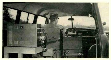
Facsimile equipment connected to two-way radio circuit produces a telegram while the driver proceeds to point of delivery. Six cars being tested in Baltimore, Md. use special radio and conversion equipment shown at left. Facsimile machine to right of driver reproduces telegram transmitted from office
