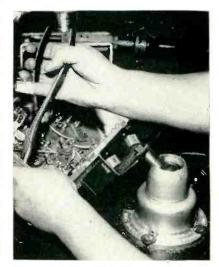
Type of holder used for gripping side of chassis. A screwdriver is required for inserting and removing a chassis. This setup is sufficiently rigid for heavy soldering and assembly work
