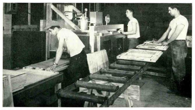
CABINET WALL GLUING—Glue used to join mounting blocks and other wood members to panels of television cabinet subassemblies are cured in about 15 seconds in this Westinghouse 10-kw installation. Man at right places blocks and strips in pallet-type positioning jig: outer panel is set over this after glue is applied
