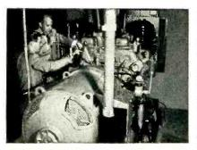
WJR—Detroit, Michigan, uses 200 kw. GM Diesel generator set as stand-by pawer for 50,000-watt transmitter. Campactness of unit permitted installation in garage adjoining transmitter building—eliminating cost of a specially designed building.
