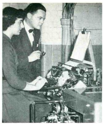
Electronic photocomposing machine used to make negatives from which an entire book, "The Wonderful Wirld of Insects", was recently produced. Housing of this developmental model has been removed to show mechanism
