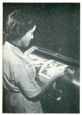
Placing original copy on Roneo stencil machine. Stencil is rolled around left-hand cylinder. Adjustable cam disks at right, acting on snap-action switches, can be set to crop top and bottom of copy
