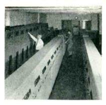
Manual forwarding units are at left, and cross-office units and multiple call processing equipment are at center and right in this view of the teletypewriter switching center
