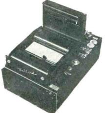
OPEN VIEW OF 708-B (8") recorder showing supply and take-up drums, operating controls.
