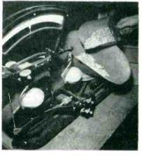
Use of ratio scale to count out 2,000 screws. The stock man previously placed 20 screws in the right-hand small pan. Scoop is easily made by nailing sheet metal to half-circle of wood and drilling hole for handle
