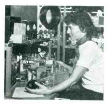
Simple instrument-grounding system at uhf test position
