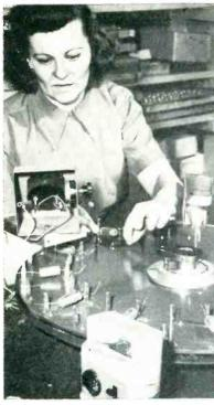
Turntable arrangement used in East Newark, N. J. plant of Astron Corp. for clearing shorts in metallized paper capacitors
