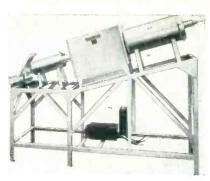
New germanium production furnace made by Hevi Duty Electric Co., Milwaukee, Wisconsin. Crank at upper left on machine is used to pull the boats of germanium oxide through the various stages of the furnace. Square center section is 1,000-deg C second-stage furnace
