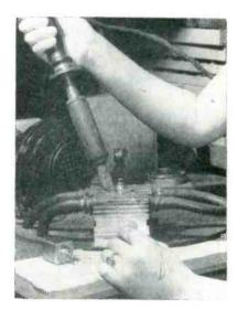
Production setup for keeping discriminator cool while making hermetic solder seal
