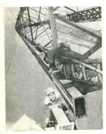
First high-power uhf transmitter uses klystron to feed television signals up 1,000-foot waveguide to antenna with power gain of 22
