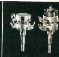
Centralab Model 2 Radiohm. Left, twin unit plain type, front section tapped; Right, twin unit switch type, rear-section tapped. Concentric shafts.
