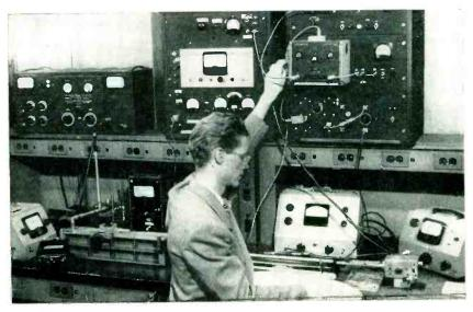
Laboratory setup of equipment used to measure characteristics of 1N72 mixer crystals
