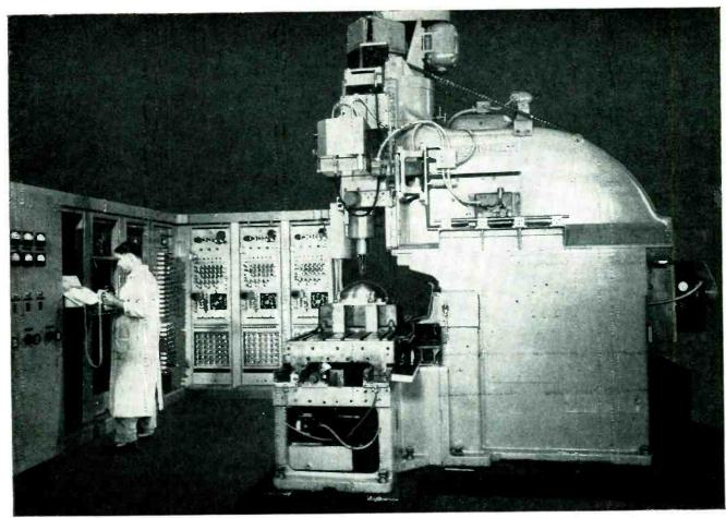
Cincinnati Hydro-Tel, automatic 28-inch vertical milling machine, is controlled by 250-tube electronic director
