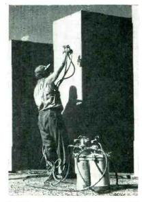
Spraying concrete blocks for cosmotron with dust-preventing resin. Preliminary tests indicate the solution also has waterproofing value
