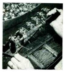
Six-unit holding fixture speeds subassembly work on television receiver controls by providing best work angle
