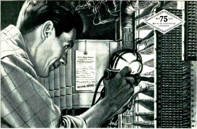
Western Electric installer in an aircraft plant connecting telephone equipment with a G-E soldering iron.
