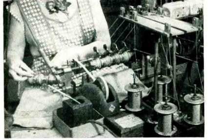
Winding flyback coils in multiples of four on keyed mandrel. Dereelers are on tops of wire spools at lower right. Tape for anchoring leads is in heavy dispenser, with end of tape anchored over tailstock so pieces can be cut easily with scissors that are always in operator's right hand. While winding is in progress, operator cuts the adhesive tape into strips and sticks them on her left hand, ready for instant use
