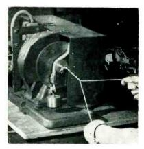
Method of using modified tapping machine for twisting leads together
