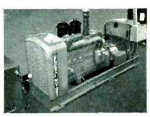
WKTV—UTICA, N. Y., uses a 100 kw. General Motors Diesel generator set for stand-by power. Set can be started remotely from the control room. Low vibration characteristic of engine permitted installation in room adjacent to transmitter and within 30 feet of studio.
