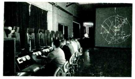
Pilots seated at a multiple console fly in accordance with traffic controller's telephoned instructions from desk at center rear. White dots on chart at right represent the craft. Simulated radar presentation on common screen is electronically controlled and viewed in mirrors above each position
