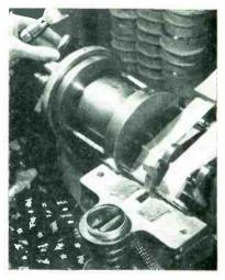
Inserting first half of split arbor along with pointed rod by pushing slide with left hand, preparatory to anchoring start of next winding so that strips can be cut
