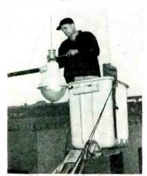
Technician installs radio control unit atop street light. Instant blackout of New York City will be possible by signal from station WNYC
