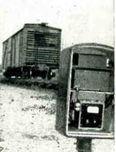
**OPERATOR** in freight-yard control tower (left) engages remote car-retarder when speed meter (right) warns that coupling speed is unsafe os . . .
