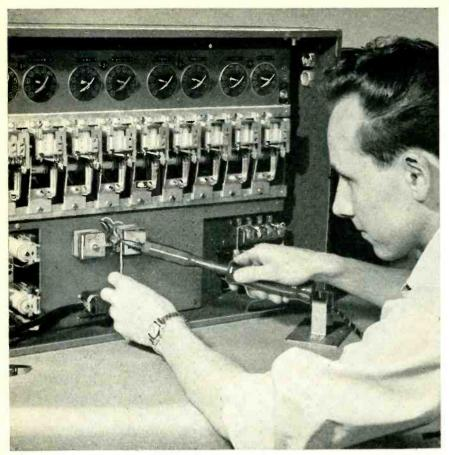
Operator installs space-saving G-E Selenium Rectifiers on monitor sequence count-controller.
