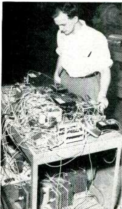
Appearance of breadboard setup for two-stage self-excited magnetic amplifier voltage regulator being designed for use in the atomic-powered submarine Nautilus
