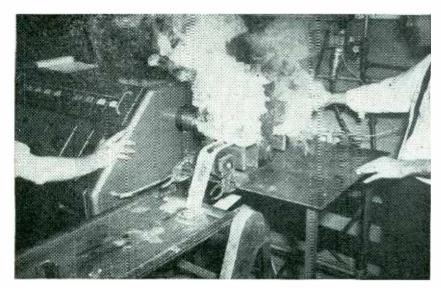
Experimental plastic preheater. Radiation through the entrance and exit holes in the cavity is reduced by quarter-wave chokes
