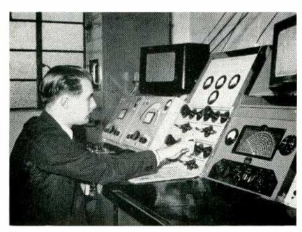
Television sound signals at audio frequency are passed to this control room for monitoring and redistribution over the feeders
