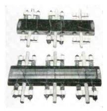
Tube-holding racks. Phosphor bronze heater-connecting strip is on one side of rack only. Strip folds over end at left. Short metal piece folded over end at right serves to connect together the strips on the two adjacent racks when they are stacked
