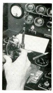
Testing 6CD6G in universal shorts and gas test set. Tube socket panel is held down by locking latch at right, needed for larger tubes. Coil spring makes top cap connection
