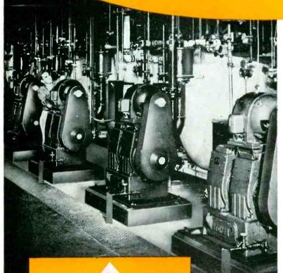
Typical installation of Stokes Vacuum Pumps.
