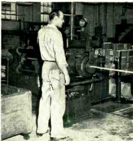
CERAMIC CORES are made by extruding refractory material from hydraulic presses such as this in Ward Leonard's plant.
