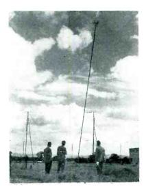
Receiving antenna on 120-ft tilted pole is positioned at focus of 220-ft parabolic reflector made of fine wires
