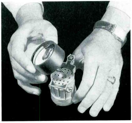
FIG. 2—Plug and flux meter setup used to make field measurements on ion traps
