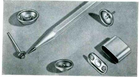
Hairline Leakers Are Eliminated in these cathode-ray tube parts and crystal cartridge components for glass-to-metal sealing. Standard Volkert items, formed to close tolerances from Allegheny HC-4 Sealmet and Kovar.
