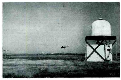
Baby VOR (vhf omnirange) in experimental use at National Airport, Washington, D. C., for approach guidance. Monitor antenna is at left
