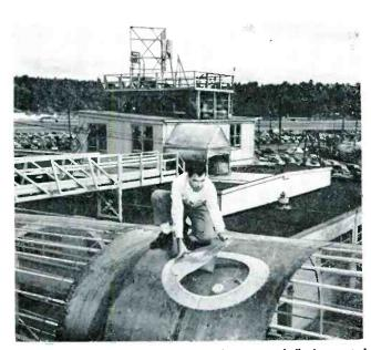
ANTENNA MOCKUP For testing performance of flush-mounted antennas, wire mesh is as effective as regular aluminum airplane skin. Boeing engineer Michael Schwartz is here fitting such an antenna on a full-size mockup of the Boeing B-47 Stratojet bomber. Structures in background check radiation patterns of scale-model antennas on scale-model planes
