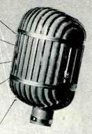
The £39B is the well known standard for directional microphones. When studio noise or other conditions dictate a directional unit, the £39B with its six selective patterns is sure to fill the need.
