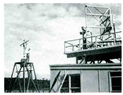
Antenna laboratory of the Boeing Airplane Company housed at right and tower at left on which model airplane is mounted for tests. Radio waves beamed from horn atop laboratory are received by model antennas inside model airplane. Signals thus received are conveyed back to laboratory by shielded cable for strength measurement as airplane is rotated
