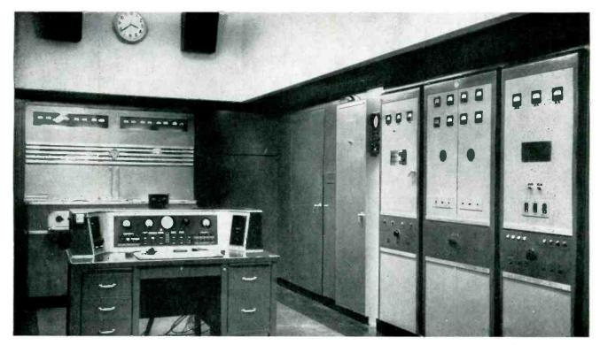
Complete emergency television transmitter with filaments lighted. In event of main transmitter failure, operator flicks toggle switch and moves chair to emergency console. Coaxial cable run starts behind false wall back of clock and continues around to right.
