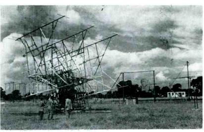
British version of moon radar is built on World War II searchlight base. Smaller type is shown at right, while in background may be seen meteor radar antennas.
