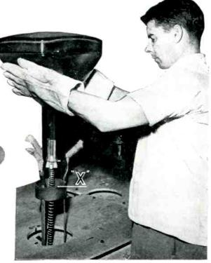
This view shows how the tube is placed on the spider which is held in place by an Inconel "X" spring.
