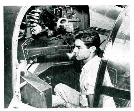
RADAR CHECK Final on-the-ground check of radar equipment in radar observer's station of Northrop Black Widow F-61 night fighter
