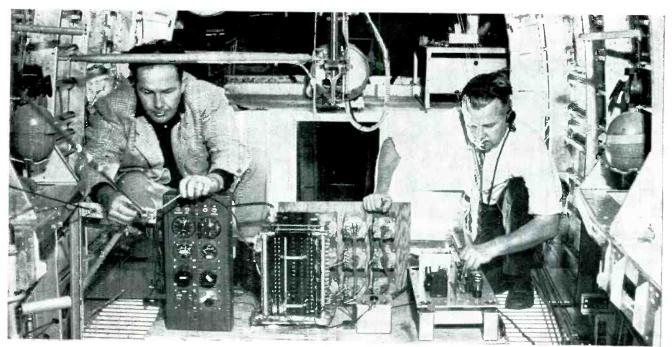
IN-THE AIR TESTS Convair electronic engineers install a pressure-survey panel and strain recorder in B-24D in preparation for flight lests that involve checking of airframe performance as well as electronic gear
