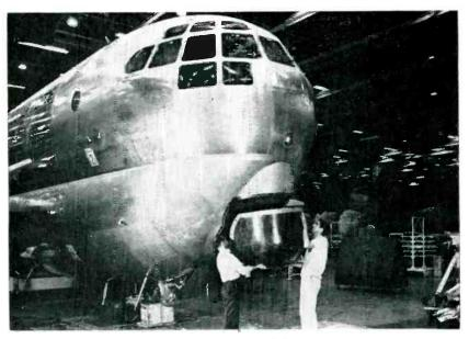
PROTUBERANCES Though still permitted on relatively slow planes such as this Boeing-made C-97 Stratofreighter, all protruding antennas and radomes are much deprecated for travel at speeds approaching or exceeding Mach 1
