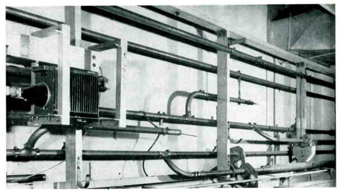
Top two lines carry f-m. Next line down is emergency sound. It passes through coax switch. To it is attached compensating stub near center of picture. Regular sound line comes in from right through another coax switch and joins extension of emergency sound line. Next lines visible are emergency picture and regular picture lines
