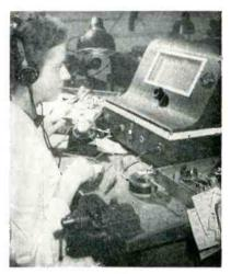
Speed of watch strokes are checked by a technician
