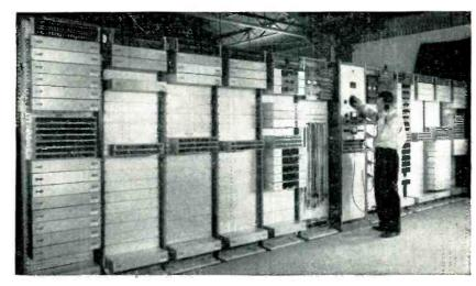
Carrier equipment racks for control station of aeronautical communications network
