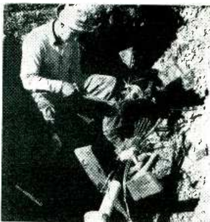
Worker makes a splice on a section of the coax cable between Pittsburgh and Cleveland, part of the link joining the Bell System's eastern and midwestern television networks. Splices are made in a temporary pit dug into the ground to the level at which the cable is placed by the plow
