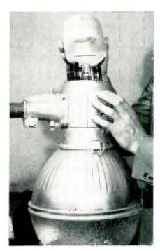
a red-sensitive gas-filled phototube, two amplifier tubes, a filament transformer, and a relay element.
