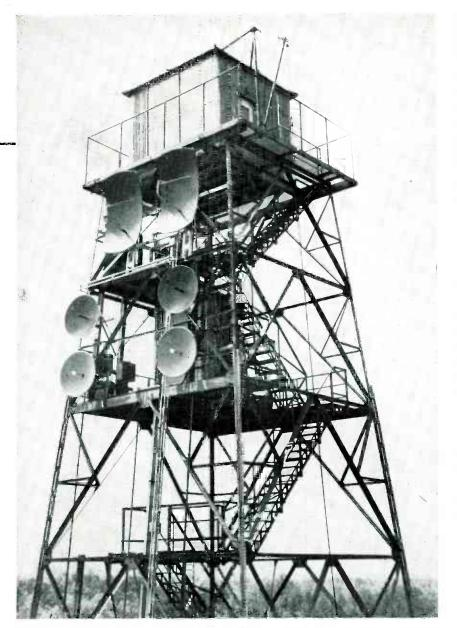
Antennas, horns, and waveguides installed on Western Union tower at Neshanic, N. J.
