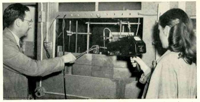
Use of radiation survey meter for monitoring hot samples during preparation of radioisotopes for industrial uses. This provides a continuous check of the efficiency of techniques and materials used to protect personnel against excessive radiation exposure
