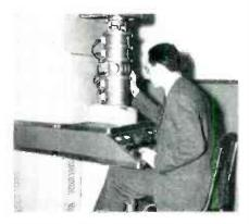
chemical composition and atomic arrangement of crystalline substances by directing a beam of electrons through a minute specimen,
