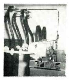
Top of cabinet installation at Neshanic, showing complete antenna switch for 6,000-mc television relay system
