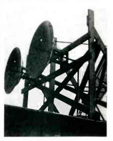
Four-foot parabolas installed on the roof of Jamaica station for beam t.ansmission and reception
