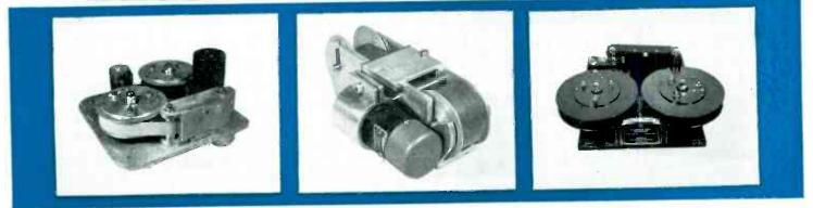
Recorder Mechanism — Type MR-2; netic Tape Recorder Mechanism — applicable to flight tests of engine Type MR-3; especially suited to temperatures, accelerations, strains, etc. guided missile applications.
