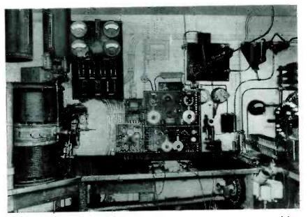
Radio room of Army transport about 1918. The 5-kw arc transmitter is at left
