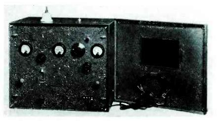
Transmitter receiver used in motor lifeboats carried by passenger vessels
