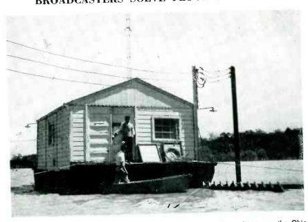
Radio station WKYW, Louisville, Ky., now has a water-borne transmitter near the Ohio River. In the path of frequent floods, it was installed on a barge and rises with the river. The barge is held by steel cables
