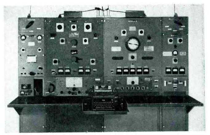
Typical packaged shipboard installation including automatic alarm (with keyer unit), high-frequency transmitter and receiver, intermediate-frequency transmitter and receiver, emergency transmitter, antenna switch, and charging panel. Motor generators are in lower section
