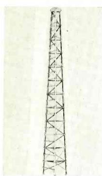
61ST aluminum alloy. Delivered knockeddown, it can be erected by one man. It is designed for low cost developments in the f-m, a-m, and television broadcast fields.
