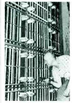
FIG. 1—Airborne particles receive a positive charge as they pass through this ionizer unit
