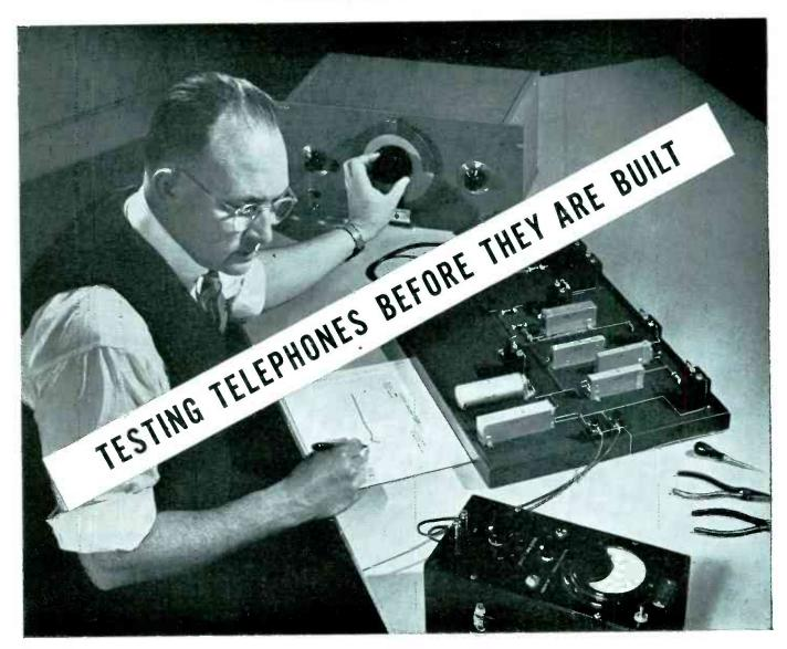
A TELEPHONE RECEIVER is a complex system of electrical and mechanical elements. Its coils, magnets, diaphragm and cap react on each other as they convert the electrical waves of your voice to sound waves. What is the best size for the holes in the ear cap? Will 1/1000th inch greater thickness help a receiver diaphragm to carry your telephone voice more clearly? One way to find out is to build numerous experimental receivers and test them.
