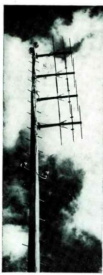
Beam antenna for 156 mc atop Yankee Network studios in Boston is used to program Paxton transmitter about 45 miles to west
