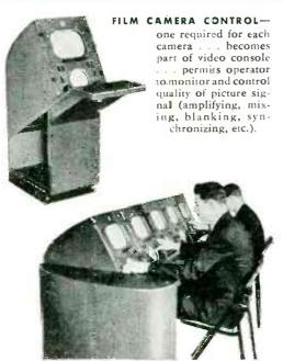
VIDEO CONSOLE—composed of studio and film camera controls, a master monitor, and switching, lap-dissolve, and fading facilities for selecting the camera pick-up desired. "Building-block" design assures a compact, unified appearance... permits adding extra units at any time.
