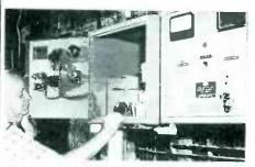
FIG. 3—High-voltage power supply for the precipitator units
