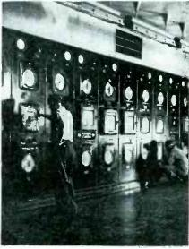
Scores of electronic, pyrometric, and pneumatic instruments are mounted on the four walls of this air-pressurized control room to direct 500 control points in the giant new catalytic refining unit built by Gulf at Philadelphia
