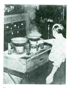
Necks of milk cans are now heated electronically without annealing the entire breast of the can and one man does the work of two formerly required in this and subsequent pickling operations
