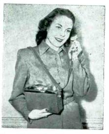
Two-way portable for the Citizens band as engineered by Hallicrafters and encased in leather, metal, and plastic
