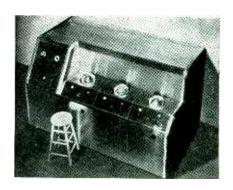
possible to keep material in various phases of the treatment. A vacuum as high as  $5\times 10^{-6}$  millimeters of mercury is quickly attained. Furnace heating is accomplished with large-diameter tungsten elements using low voltage.
