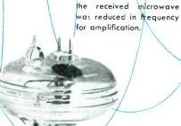
1937. This microwave generator, the 368A, was the first commercial tube to generate frequencies higher than 1500 mc. This type of tube was used by Western Electric in the first absolute altimeter.
