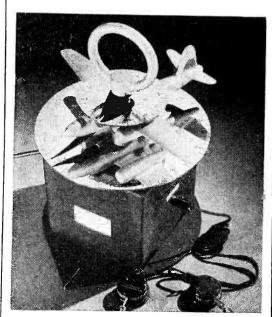
airplane in relation to the North magnetic pole and the setting of the radio loop antenna combine to indicate a bearing from airplane to station. All of the elements are movable in order to set up different problems.
