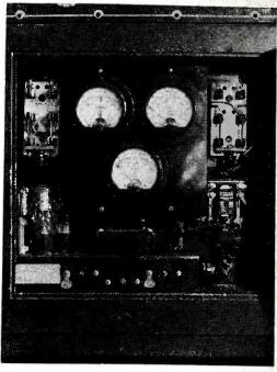
A constant d-c supply to a rotary converter from the unit above provides a stable a-c voltage for critical equipment
