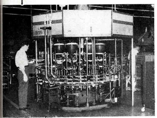
As tubes index at stations in this machine, the electrodes are inserted, flares and bulbs are sealed, and their cullets are cut off, all automatically. Various patterns of gas flames perform these operations at the Lancaster, Pa. plant of RCA Victor while the overhead hood draws off combustion products and heat
