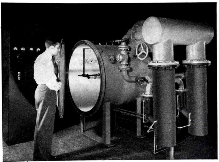
This High Vacuum Coating Unit is designed for low-cost production of evaporated films on glass and plastics.
