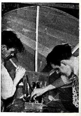
Lighthouse tube oscillator, mesh screen parabolic reflector, and tomato can bottom reflector used by George H. Floyd W60JK/2 and Arthur R. Koch W9WHM/2, General Electric engineers, in first two-way contact
