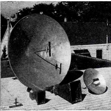
Pyramidal horns and parabolic reflectors for covering frequency range from 500 mc to 10,300 mc to provide required wavelengths for scale model antennas
