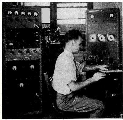
Microwave transmitter rack (left), audio and synchro control rack (right), and antenna pattern recorder used in conjunction with model-supporting tower and antenna outside
