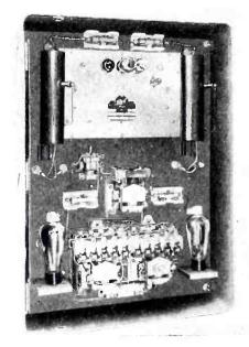
from a-c power have been announced. One model is a general purpose, reversing type applied to a 2 hp, 230 volt d-c motor, and the second is a special control for an abrasive surface grinder. For any speed setting, performance is practically equal to that of a synchronous motor even with a suddenly applied load.
