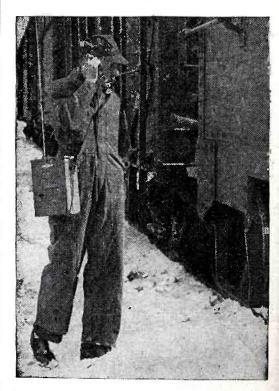
Track-side railroad crewman communicates with conductor over two-way handietalkie developed by Bendix engineers
