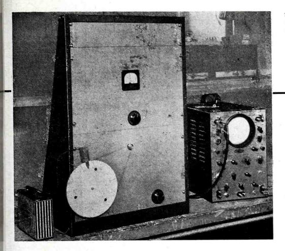
Sweep-frequency receiver and associated monitor scope. Receiver and motor drive on lower chassis, with d-c amplifier and motor control circuits above
