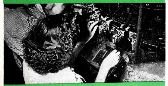
GLASS HEADERS. Small cylindrical cups of glass and metal pins are pressed into the low-loss glass base to which is joined the small glass exhaust tubing.
