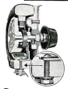
The sturdy screw terminals are integral with the massive ceramic winding core—a great core that gives 25% more capacity. These solid screw studs cannot be deformed nor ripped loose.
