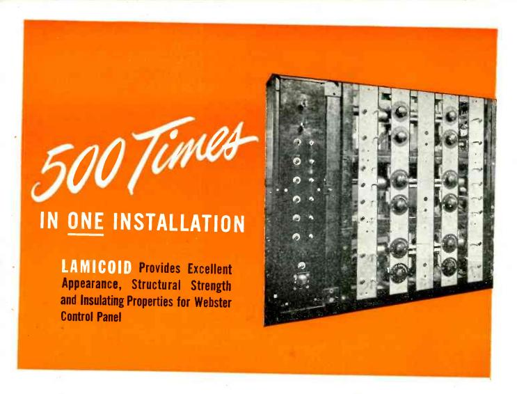
Over 500 pieces of Lamicoid help special-made Webster "Moderator" Control Panel provide automatic heat variation. Front and rear views of this 37-zone installation reveal the use of this thermosetting plastic laminate for dials, washers, and terminal boards.
