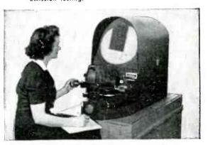
Comparator measuring dimensions to 10 thousandths of an inch, for inspecting the quality of work going into electronic tube calhodes and parts. This is just one of many tests conducted by the "Quality Control Group" of the Superior Laboratories.
