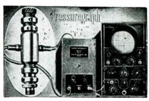
sired. Covers wide range of engine speeds and pressures up to 10,000 p.s.i. Screws into cylinder and can be calibrated using static pressures. Vibration-proof. Accurate, dependable for frequent engine tuning. Simple operation — only one control.
