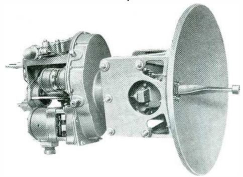
At the close of hostilities Dalmo-Victor was producing and delivering nearly 90% of the night fighter Radar Antenna-Scanners used by the U. S. Navy. We had developed the top quality product in this field.
