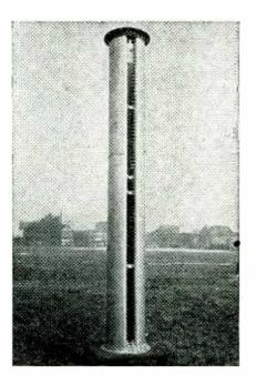
is 13 feet high, with a diameter of 19 inches, and weighs 350 pounds. Each end is provided with a flange for mounting on a base, display of a beacon at the top, or addition of another element. Radiation is horizontally polarized.
