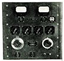
ously variable from 50 cycles to 50,000 cycles in four ranges. Accuracy of the Q measurement is approximately 6 percent.
