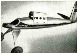
P-K binding head Type "Z" Screws fasten cabane to fuselage. Slots permit wing assembly to be moved back when model is changed over from "Class B" to "Class C", with heavier motor.
