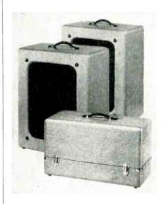
uses a 30-watt amplifier and two 12-inch speakers. Weight of the Model KX-30R12A equipment is 147 pounds.
