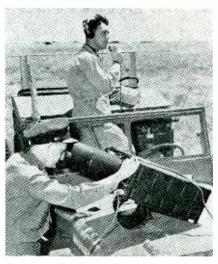
Practicing for the atom bomb tests at Bikini, Captains Davis and Seldomridge direct the takeoff of a pilotless B-17. The television receiver in the foreground shows the instrument panel of the bomber while the small control box is used to direct the takeoff and landing. The mother
