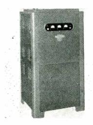
purpose unit suitable for both induction and dielectric heating operations. Full load output is about 285 Btu per minute or 5 kilowatts. The induction generator operates on 375 kilocycles and the dielectric on 20 megacycles. Changeover from one method to another merely involves replacing one radiofrequency unit with the other.
