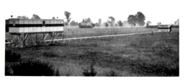
CAA instrument landing installation at Indianapolis. Antenna building is at left, in line with the end of the runway, while transmitters are in smaller building at right and 300 feet away
