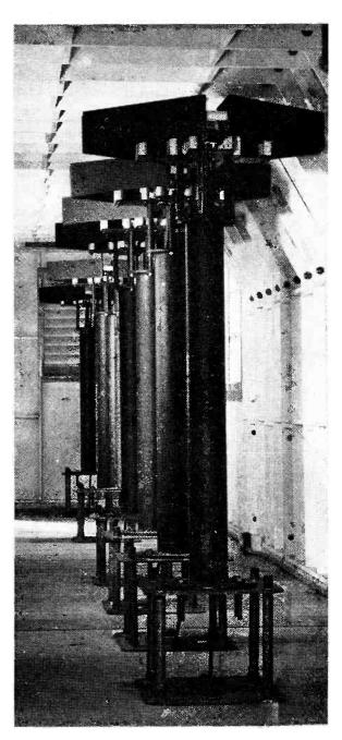
Inside of antenna building, showing array required to produce a straight localizer course. Technical details of this system were given in the February and March 1945 issues of ELECTRONICS
