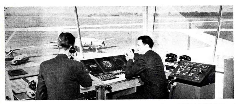
Airport control tower at Indianapolis, used by CAA in testing electronic aids to aviation. Control panel at right monitors performance of instrument landing system, and cabinet just barely visible at left houses radar scopes
