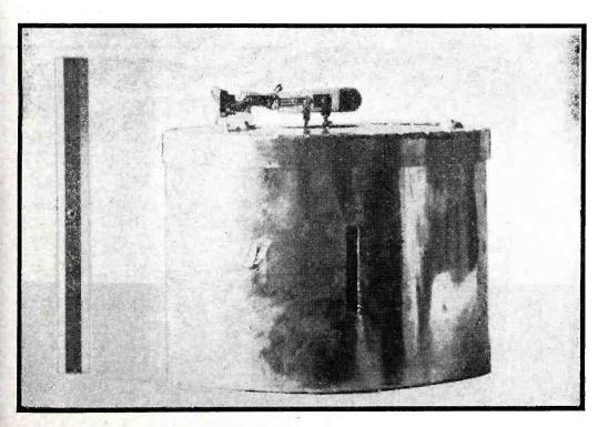
Uhf oscillations are obtained from negative-grid triode by inserting the transmission line tank into a cavity resonator
