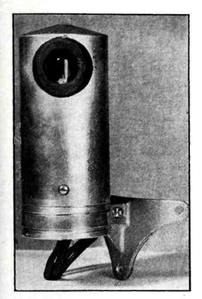
Sunswitch suitable for mounting on a street lighting system pole
