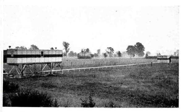
CAA instrument landing installation at Indianapolis. Antenna building is at left, in line with the end of the runway, while transmitters are in smaller building at right and 300 feet away
