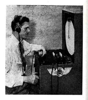
Flight-path recorder and automatic radio range of the Curtiss-Wright Dehmel electronic flight trainer for embryonic pilots
