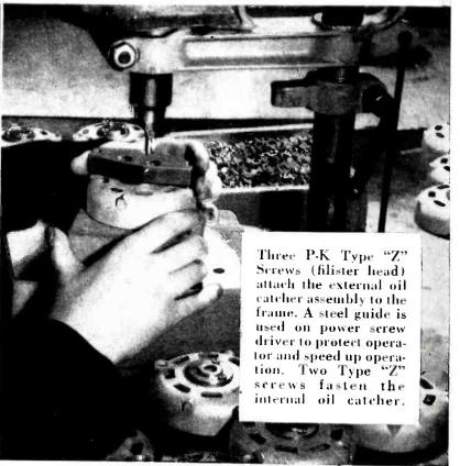
The Redmond Company Inc., of Owosso, Michigan could have assembled MICROMOTORS with machine screws. But Redmond design engineers wisely questioned fastening methods before assembly operations were started. Their conclusion: "It was obvious that P-K Screws would be less expensive to use." Why? Because seven time-consuming tapping operations in each motor could be avoided, tap breakage eliminated, and spoilage reduced to a minimum.
