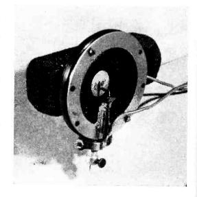
Mechanical arrangement of needle assembly and diaphragm mountings on the carbon-button pickup
