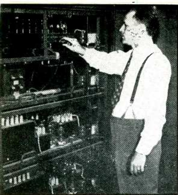
Herbert Kaufman adjusts the bias on the high-level multiplying stages of the transmitter. Kaufman and the four others shown were the personnel of "project Diana"
