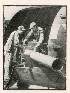
Field wire may now be laid from an airplane by means of apparatus such as this, shown being installed in an Army C-47. The splice detector is particularly valuable in checking such wire, since discontinuities are frequently masked by insulation
