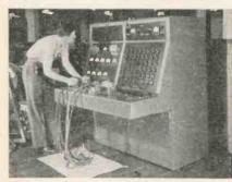
Above is the front view of the Universal Test Unit that preheats all tubes except rectifier, short tests all tubes (each element separately), noise tests RF and AF tests, static tests all tubes for all characteristics except plate resistance and amplification factor, dynamic tests mutual conductance, gain and power output at 400 cycles.
