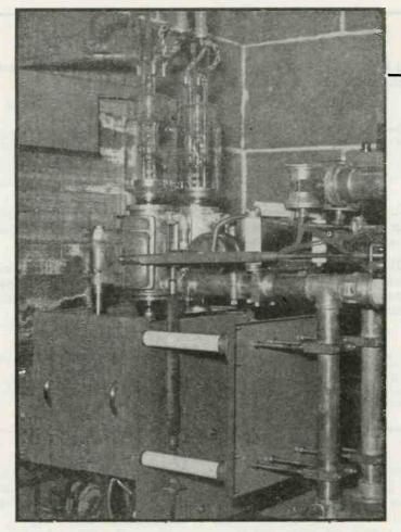
The 50-kw final amplifier at WMFM, using a pair of WL-899A tubes. Filament circuits are at the top, grid circuits at the bottom. Neutralizing capacitors are built around the tubes. The tuning capacitor and part of the tank circuit can be seen
