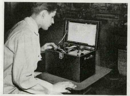
TIME-SAVING carbon content analyses of steel samples—from molten metal to report—take only five minutes with the portable, *battery-powered* Carbanalyzer, produced by the Fisher Scientific Company. Leading steel firms employing open hearth or electric furnaces quickly make carbon determinations of each steel batch, achieving close control of quality.
