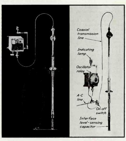
Typical industrial application of oscillator relay system, as installed in a fuel tank to sense the interface level between water at the bottom of the tank and gasoline above the water, and photographic illustration showing component parts of this installation. The oscillator relay here controls a pump that removes the water from the bottom of the tank when it rises above a predetermined level
