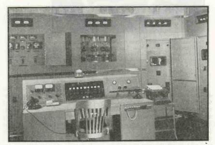
The WMFM control room. Units, from left to right, include the 250-watt r-f amplifier and modulator, the 3-kw amplifier, the 15.000-volt. 7.5-ampere rectifier and the low-voltage control equipment. The master-control console is in the foreground
