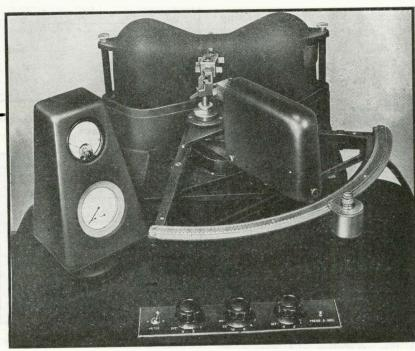
Focusing spectrometer engineered by North American Philips Co. The counting meter scale at the lower left indicates radiation intensities directly as the Geiger tube is rotated from one end to the other of the graduated quadrant that shows diffraction angles. The x-ray tube is in the dumbbell-shaped housing at the rear
