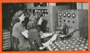
QST-2—A unique test is applied to every United tube to assure noise-free operation.
