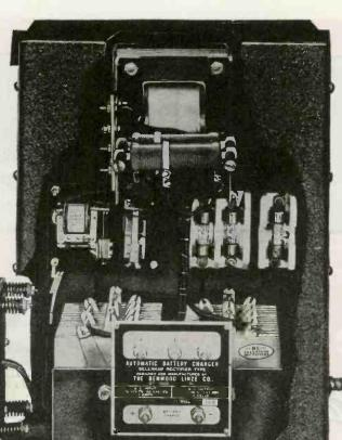
At left—Another example of B-L. Battery Charger designed to meet specific needs.
