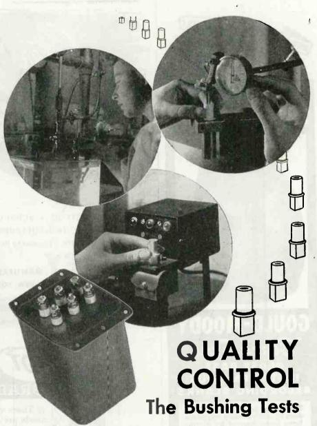
The maintenance of uniformity and accuracy in component parts is a recognized prerequisite of quality in a finished transformer, as in any precision product. For this reason, important parts of Chicago Transformers are closely inspected and tested for structural and dimensional accuracy before they reach production.
