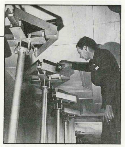
Checking adjustment of loop antenna system for runway localizer of newlyadopted CAA radio instrument landing system
