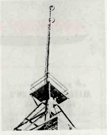
A new two-bay General Electric circular antenna was recently installed by Columbia Broadcasting System engineers atop the 700-ft building at 500 Fifth Avenue. New York City for use by station WABC-FM. Provision has been made for adding two more bays to this 14-ton structure, the height of which is 100 ft above the roof. When the antenna is put into use, CBS will have the first f-m station in New York City to
