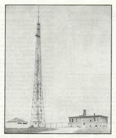
WMFM transmitter building and antenna at Richfield, Wisc. The tower is 200 ft high, and on top of it is a two-bay turnstile. The platform at the 175-ft level supports a studio-to-station link receiving antenna. The elevated trough carrying two coaxial transmission lines between transmitter house and tower may be seen
