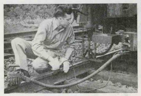
When a rail is suspected of having a defect, white point is sprayed from the moving car on the tracks. As shown above, an additional test probe of the electronic equipment is then used to find the exact location
