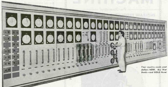
When war called for greatly increased supplies of industrial alcohol, installation of this control panel helped a midwestern distillery to step up its production of high-proof spirits. These control instruments made possible the quick conversion of a low-proof distillate tower to production of 190-proof alcohol.
