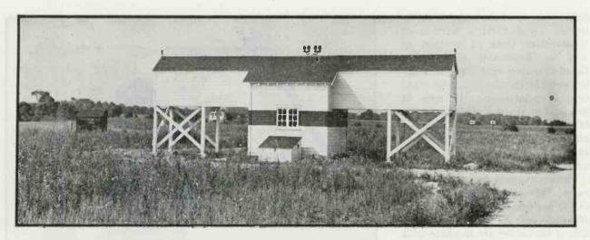
Building housing runway localizer antennas and associated transmitter equipment
