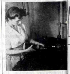
After soaking in warm water for 1 hours, cathode-ray tube bases are inserted in the holder shown above and the tube twisted against the torque of the weight on the arm. Virginia Connick tests the cement on the tube base in this manner at the Dobbs Ferry plants of North American Philips
