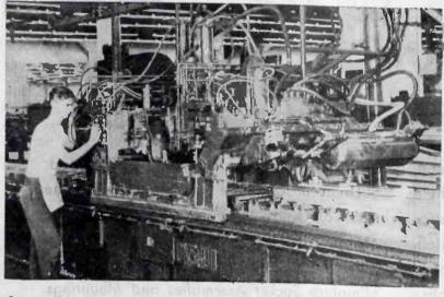
Automatic contour milling machine in operation. Equipped with G-E Thy-mo-trol. it does in 5 minutes a finishing operation in the machining of aluminum spar beams that formerly took 13½ hours
