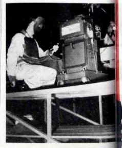
To insure safety in flight, duralumIn spars of the extensive wing section of a Clipper are x-rayed for possible hidden flaws that escape visual inspection
