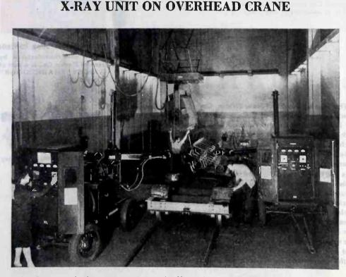
Crankcases and other component parts for Navy ships are x-rayed for possible faults at Warren City Mfg. Co., Warren, Ohio. One of four of its kind in the country, the overhead x-ray equipment in the background can photograph steel plate up to 4 inches thick. Other portable industrial x-ray units appear in the foreground and extreme background
