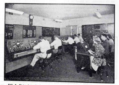
FIG. 3—Main shore station at Lorain on Lake Erie. Each of the six operator positions has push-button selection controlling six transmitters and receivers
