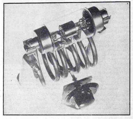
Tank circuit utilizes vacuum capacitor of Eitel-McCullough design. Internal construction features rigidity for the maintenance of stable capacitance values
