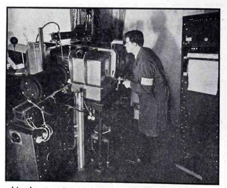
Infrared spectrograph used in Socony-Vacuum Laboratories. The spectrograph proper is in a metal housing to permit evacuation for removal of water vapor and carbon dioxide. On the rack at the right is the pen and ink recorder that traces out the spectrum of the material being analyzed
