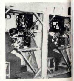
Separate cubicles simulate the radio room of a plane and help train RAF signal cadets to find troubles in radio equipment under crowded conditions
