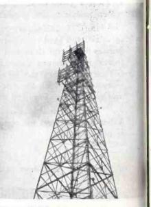
Two parallel arrays of half-wave elements mounted 200 feet high form each antenna in the radiotelephone link across Chesapeake Bay
