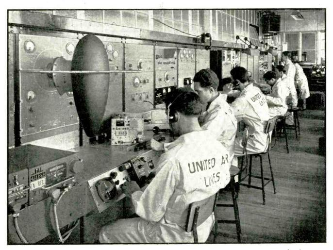
Test panels in the radio-electric department of United's base in Cheyenne. Left to right: Automatic direction-finder test panel; receiver test panel; interphone and loop test panel; oscilloscope for visual checking; a-f signal generator and vacuumtube voltmeter; communications unit test panel; a.f power amplifier; loop gear box test panel; all-wave receiver for checking frequencies; microphone and headset test panel; autosyn test panel; relay test panel; generator test panel
