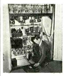
A technician checks some of the electronic equipment used to control the speed of a 24-foot fan in America's fastest wind tunnel. It produces gales of 700 miles an hour, almost equal to the speed of sound, and was dedicated by Boeing Aircraft Co. as the Edmund T. Allen Memorial Aeronautical Laboratories in memory of the test pilot killed last year
