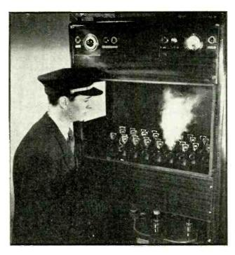
Numbered pipe outlets in the smoke-detecting cabinet show the ship's officer at a glance which space is afire when the photoelectric cell sets off the automatic alarm in the Rich-Audio fire-detecting system made for ship use by Walter Kidde & Co., Inc., of New York
