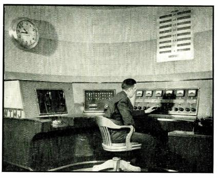
Master control room from which circuits may be set up in advance at Radio City
