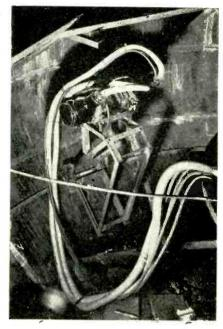
The head of the x-ray tube was mounted down inside the reacter for examining the welds in the lower conical sections. A monorail carriage runs on a track parallel to the weld seam
