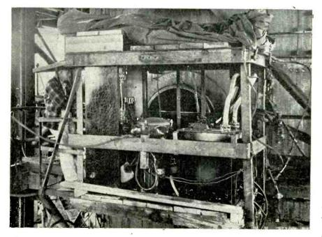
Transformers and other units of the x-ray machine were stripped of protective covers to reduce weight. The only protection against the elements is the tarpaulin shown rolled up atop the suspended crib
