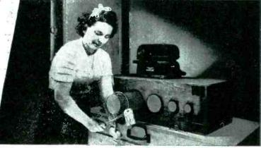
By a dozen different searching tests Amphenol RG Cable is proved before it is shipped.
