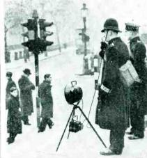
To cut down traffic accidents, British police use this portable electronic megaphone at crossings to direct pedestrian traffic. Tubes and batteries hang from the tripod assembly
