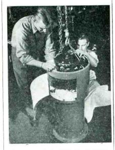
The lightweight electronic gyro-compass is fitted into its binnacle
