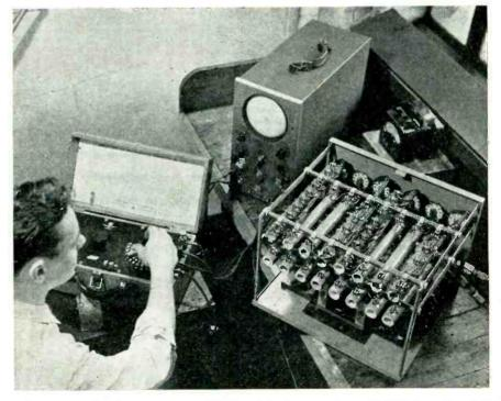
One of the circuit drawers of a calculator for a-c networks is checked for accuracy by means of a special bridge and an oscilloscope
