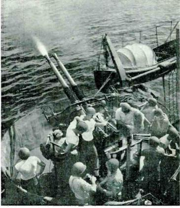
Range information for anti-aircraft guns is transmitted by inter-ship phone from control stations. The pointer, seated on gun mount at left, adjusts for elevation while the trainer, seated at far right, maintains horizontal position on the target
