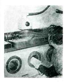
Aircraft radio instruments are tested in this cold chamber at 65 deg below zero at the radio division of Bendix Aviation Corp. Flexible coverings over the portholes of the chamber permit the muff-covered hand of the operator to adjust the controls of the equipment
