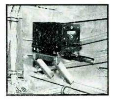
Location of amplifier unit for No. 3 engine in a B-24 airplane
