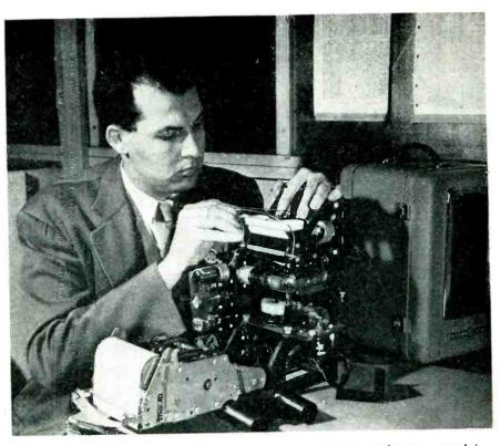
The photoelectric recorder that has a response speed of five cycles per second is tested by D. F. Hang, engineer in the General Engineering Laboratory of General Electric. Miniature mirrors and lenses are used to relay the impulses being recorded
