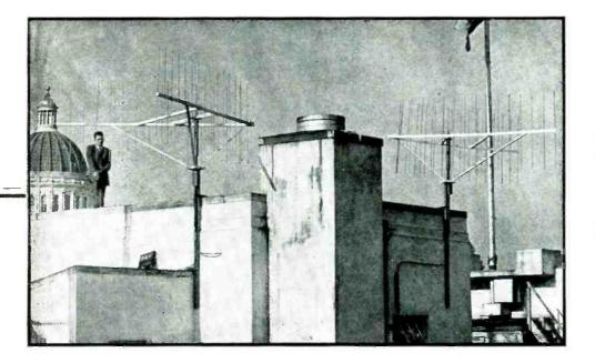
FIG. 2—The two receiving arrays on a Sacramento rooftop. Since the photographs were taken, the array at the left has been moved along the wall to the left to decrease absorption of the signal received from Mt. Diablo by a nearby vertical antenna
