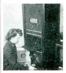
Patients at the St. Albans Naval Hospital on Long Island are entertained 10 hours a day from this Stromberg-Carlson control cabinet, operated by Lucille Ingebretson, pharmacist 2C. It contains FM and AM receivers, an automatic record changer, pre-amplifier and monitor speaker, and supplies 12 booster amplifiers on the system
