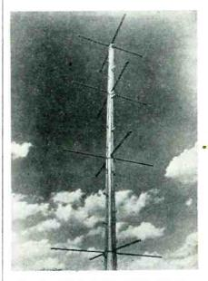
The four bays of this turnstile antenna at the Zenith FM station WWZR are fed by eight Andrew 1%-in. diameter coaxial cables. These lines and the 41%-in. feeder from the transmitter are maintained under constant gas pressure. Made by Andrew Co., the cables are connected back to back to provide a balanced 140-ohm line
