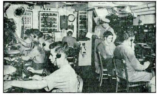
Men in the communications center maintain contact with other ships of the fleet and bases by radio and handle the inter-ship phone system. During the shake-down cruise, the crew learned how to operate equipment under combat conditons
