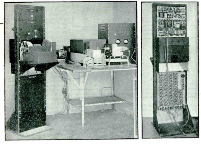
Overall view of calibrator, showing frequency meter on jig at right center, with dial coupled to zero beat detector. Printing rack is at left. Signal source is not shown
