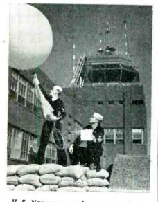
U. S. Navy aerographers mates release a weather balloon with radio sonde equipment that will transmit signals indicating temperature, humidity, and air pressure at various altitudes. Official U. S. Navy photograph
