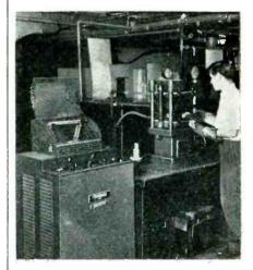
The high-frequency generator at the left is used to heat preforms at the Plastics Industries Technical Institute in Los Angeles. It preheats one pound of compound per minute before molding in the compression press at the right. Made by Airtronics Mfg. Co., a division of Aerocrafts Corp., the unit is of value in research development and practical training of students
