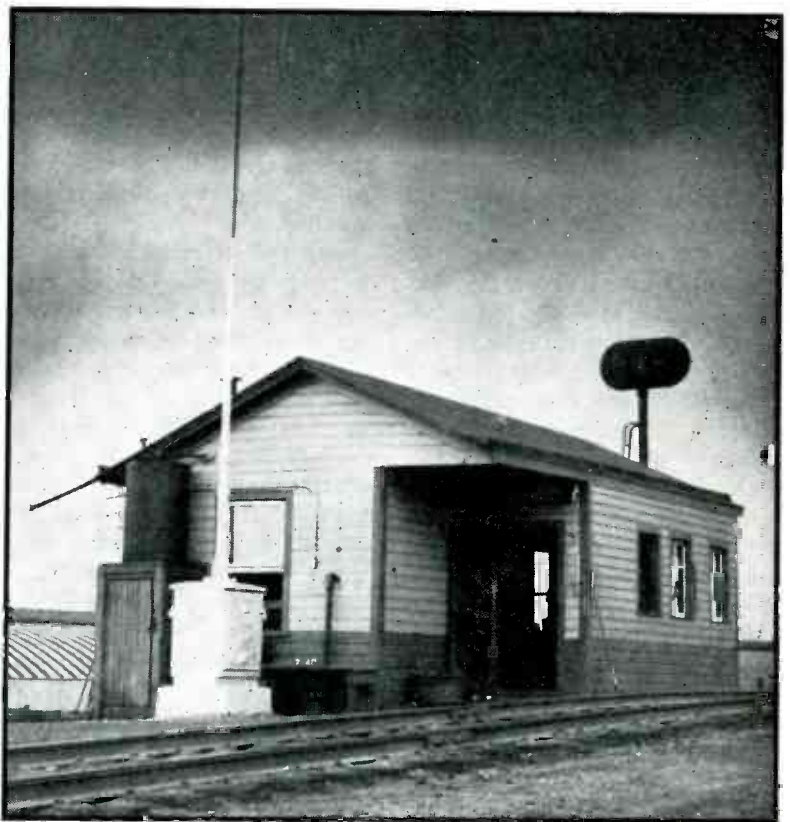
Central-station radiotelephone equipment at the "hump" in Proviso yard, developed by Halstead engineers for the General Railway Signal Company. Units of this general type are adaptable for installation along main-line trackage in radio-repeater or secondary-station services
