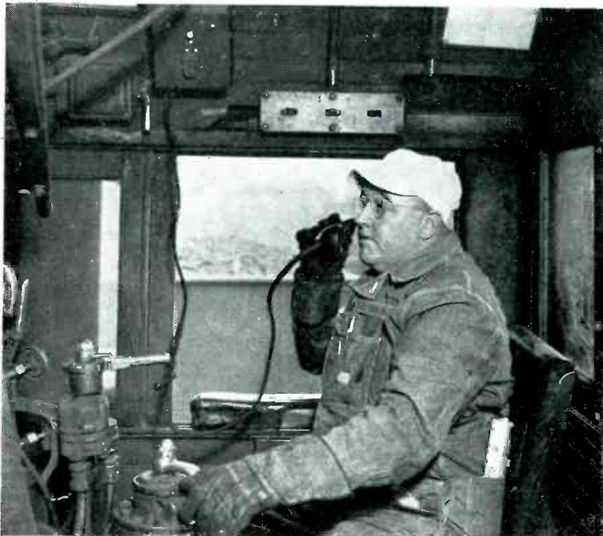
A handset with a press-to-talk switch and an overhead speaker (not shown) is used by the engineer in the locomotive cab. The carrier-current equipment, mounted above the driving wheels, utilizes the tracks and adjacent wire lines for reception and transmission from train to train or to the block operator
