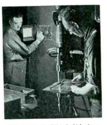
Spot-welding two .062-inch thick pieces of aluminum with 48,000 amperes of current. The ignitron welding control in the background allows the current to flow for eight cycles in this application and permits adjustment for spotwelding various other thicknesses of metal
