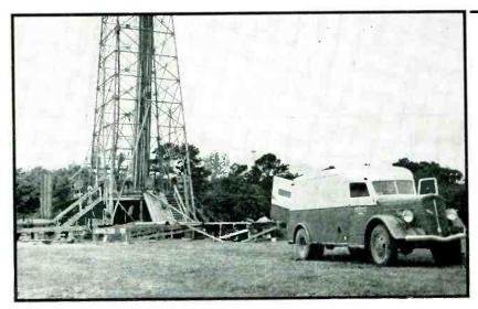
Truck set up for making an oil well log (Halliburton Oil Well Cementing Co.)
