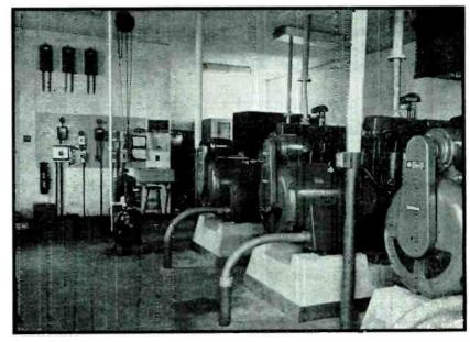
Generating plant at WMIT transmitter site, Clingman's Peak. Three dieselelectric sets generating 75 kw apiece are used
