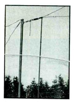
Close-up of the receiving rhombic, showing the feed-line end at which the quarterwave transformer section encased in a copper pipe and the concentric line discussed in the text are used
