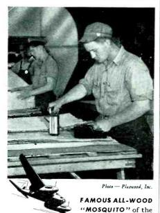
of tough, durable wood veneer — made to a rigid engineering specification. The physical characteristics of this veneer must be as uniform as metal. Most vital step in production is the drying where precision control of moisture content assures its stability and strong cell structure... guarded by electronic moisturemeters powered by Burgess batteries.
