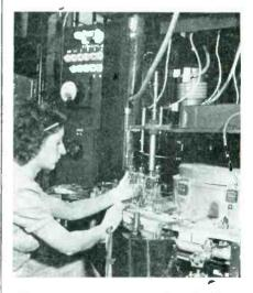
More than a dozen heating, baking and pumping operations are undergone by vacuum tubes during a 20-minute trip around this automatic exhaustion machine. Westinghouse engineers report that only one out of every 1.520,000 molecules of air or gas, present in the tube before exhaustion, remains when the tube is finally sealed
