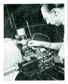
An operator checks the temperature of a hydrogen flame used in conjunction with a punch press to form glass jewels for meters. The glass rod is fed into the press by the motor drive in the foreground
