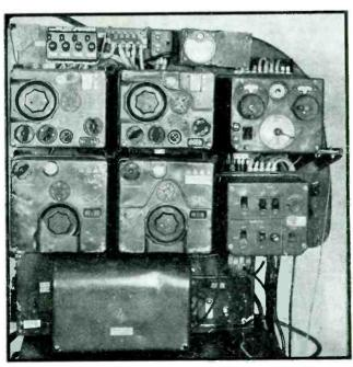
FIG. 1-The FUG-10 panel with all units in place
