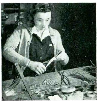
Inexperienced operators can make perfect Indent connections right from the start, and from three to ten times faster than by the older soldering methods. Absence of acid, which frequently causes finger burns, also makes job cleaner and faster.
