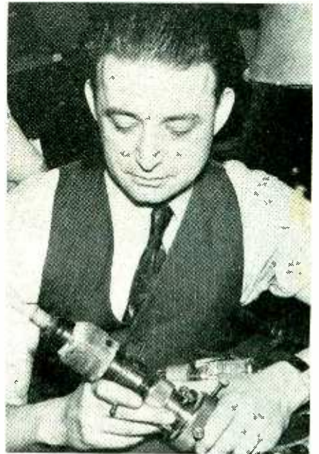
Lawrence Handler and the machine tool fixture he redesigned to eliminate breakage of vacuum tubes during assembly. The new fixture saves critical materials as well as nine production hours daily
