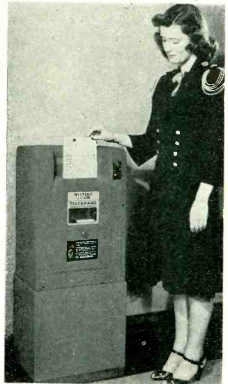
Automatic transmitter for facsimile telegraphy. The square, black block on the message blank synchronizes the scanning drums
