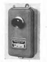
is rated up to 32 candle-power; model No. 18-B comes with a transformer and operates directly from 110 volts, a.c. Model 18-B is provided with taps to permit operation at various light intensities. It is rated up to 50 candle-power.
