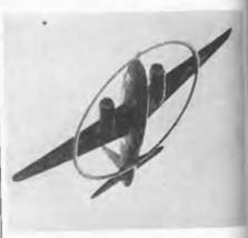
The minesweepers of the air are equipped with a hoop-shaped casing extending all around them and secured to their nose, wings and tail. The casing holds a magnetic coil and current is supplied by an auxiliary engine. This equipment was designed to set up a magnetic current which would set off the mine. The crews are severely jolted when the mines are exploded
