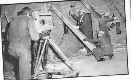
DEMOLITION-Experts show distant defense workers how best to prop up a shaky wall and handle dangerous trailing electric wires
