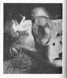
Gamma rays generated by Westinghouse electronic equipment detected air bubbles in this steel turbine cylinder casting. Flaw areas were chipped out and the man at work is filling in these areas by means of a welding technique
