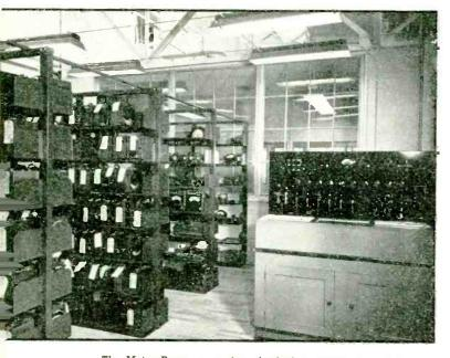
The Meter Room, a portion of which is shown here, has complete facilities for calibrating the three thousand different meters which are available for the measurement of voltage, current, power, temperature, speed, and other physical quantities
