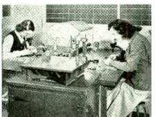
Sodium light is being used in several important war plants for surface inspection by microscope, because of its efficiency in the detection of pits, cracks, and flaws in materials. The sodium lamp is essentially an arc lamp, and differs from the incandescent in that it requires a special socket and individual control for each lamp. The unusual perception of detail under sodium illumination is due to the monochromatic nature of the light
