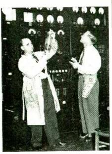
It is necessary to get every possible hour of efficient life from the giant transmitting tubes and other equipment at the 50,000 watt transmitter at KFI in Los Angeles. Frequent meter checks and constant surveillance of every circuit at the transmitter will help do the job. The co-chief engineers H. L. Blatterman, left, and Curtis Mason are shown replacing one of the big 849 vacuum tubes whose filament electron emission is no longer satisfactory
