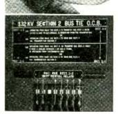
(Abore) FUNCTION AND OPERATION of controls explained in detail with Engraving Lamicoid panels to minimize misunderstandings and mistakes.
