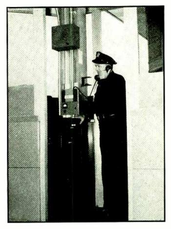
TOLL BOOTH CONTROL—Each booth, at every interchange, can listen and talk. The meter is an r-f indicator, included to make doubly sure that two or more ticket collectors do not modulate the repeater-exciting 37.5 Mc transmitter at their interchange at the same time
