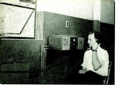
TUNNEL PORTAL REMOTE—This unit contains a speech amplifier and an audio amplifier and speaker. It is connected through a cable paralleling a 220-volt, a-c line (direct, or via the other tunnel portal) to the repeater station high overhead. Power and control and modulation currents go up. Output of repeater station receivers comes down. The meter is a modulation level indicator
