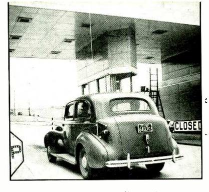
TWO-WAY TURNPIKE CAR—The halfwave whip type antenna serves a 37.5 Mc amplitude modulated transmitter exciting any one of the system's six mountain-top repeater stations (and the "shuttle" transmitter at The Midway) and a 33.94 Mc receiver tuned in on frequency modulated transmitters at four of the hills
