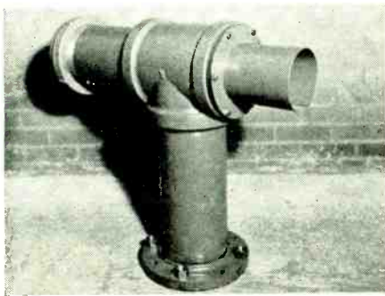
Fig. 1—Outdoor modulated light beam projector
