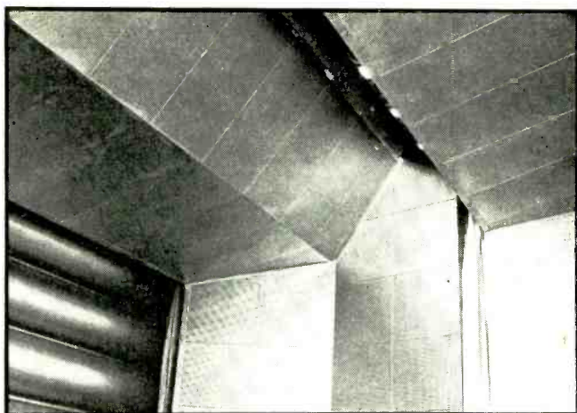
(Below) A corner of the stage showing details of the perforated asbestos board and the hard, rounded surface at the rear of the stage used to disperse the sound waves rather than to absorb them or to reflect them to some point in the studio space where they might upset the acoustic balance or be otherwise annoying
