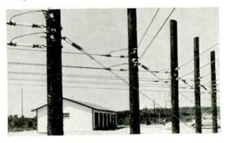
(Below) SPECIAL FITTINGS used on Isolantite strain and other types of Isolantite insulators at the new stations were designed and tested by engineers of Mackay Radio and Telegraph Company and the Columbia Broadcasting System. These fittings were manufactured by Burndy Engineering Company.
