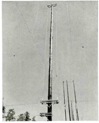
(Abore) CONSTRUCTION DETAILS of the antennas are shown here. Horizontal wires at left near base of pole provide means for tuning the antennas through the medium of variable line shunts.
