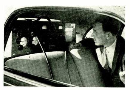
Fig. 1—The field intensity recorder is shown installed in an automobile. The recording mechanism is at the far right
