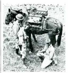
Soldiers of Troop B of the 107th Cavalry Regiment of Ohio sending and receiving radio messages using a portable pack radio set at the recent army maneuvers in Arkansas. This equipment can be used on the ground as well as on the pack and has a range of from 25 to 50 miles. It weighs approximately 170 pounds
