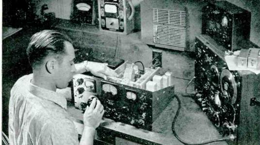
On arrival at the factory, all components are inspected and checked against the laboratory specifications
