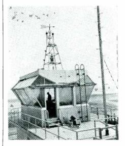
The glass inclosed tower atop the airport building at Washington, D. C., provides an angle of view of 360 degrees for directing the traffic of planes into and out of Washington. The station is also used as a local weather bureau
