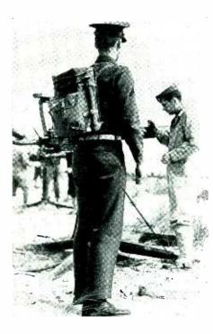
Soldier carrying Walkie-Talkie radio apparatus, used by the 62nd Coast Artillery during fire practice at Fort Tilden, N. Y., in which 50-calibre guns were used. By means of this portable equipment, two-way voice conversation can be carried on between observer on the ground and plane which tows an aerial "sleeve" target for gun fire α
