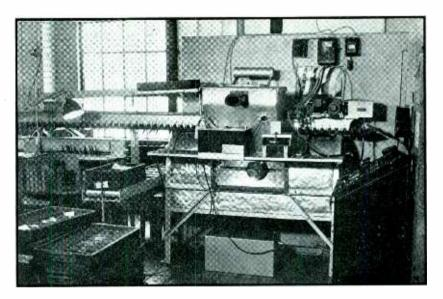
Equipment used to test an interior lead soldered joint in table knives by means of x-ray gas ionization. The x-ray tube is shown beneath the bench and the knives to be tested pass through an opening to a ionization chamber. The amount of lead in the joint determines the degree of ionization of the gir in the chamber
