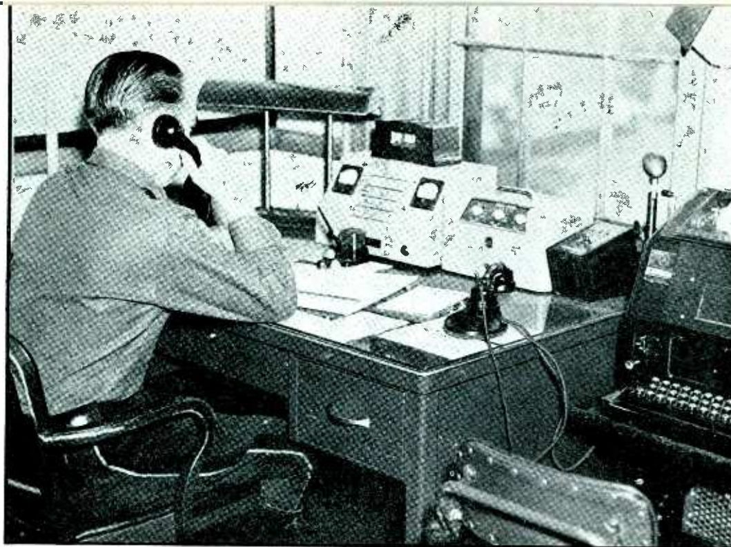
Fig. 10—The control unit at headquarters. The transmitter is put in operation when the operator pushes a button on the handset. Transmission occurs on 39,500 kc, reception on 39,180 kc
