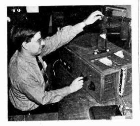
Charles Millikan, graduate engineer at the California Institute of Technology, pops corn in a cellulose bag by using short radio waves. The device operates on the same principle as that employed in diathermy machines, but is rather uneconomical when used solely for corn popping
