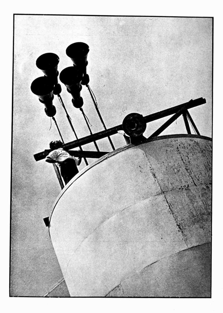
**Sound** . . Experimental 100-watt loud speakers on test during early days of New York World's Fair construction. In spite of steam shovels and other noise making machinery, the battery covered an area of <sup>1</sup>/<sub>2</sub> mile radius
