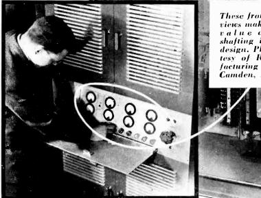
These front and back views make clear the v a l u e of flexible shafting i u r a d i o design. Photos courtesy of RCA Manufacturing Co., Inc., Camden, N. J.
