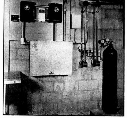
Fig. 7—A neat gas-filling installation, at WKBN. Note that a duplicate cable is maintained as a spare (Communications Products)
