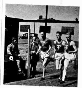
A group of track men testing out an electronic device invented by George Dadakis of the Massachusetts Institute of Technology. The track is divided into four points, at each of which a post is erected. As the runner passes the post, a bell rings. It is expected that by this method, the runner may time himself better on each lap
