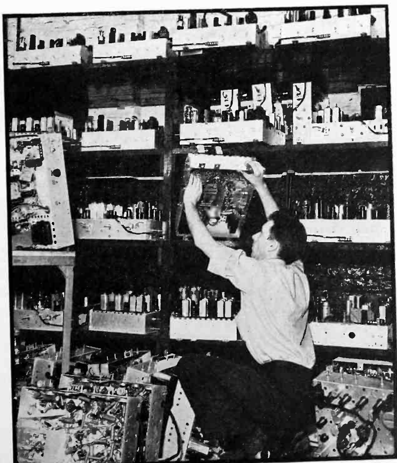
The completed chasses are inspected and placed on storage racks, ready for mounting in the cabinets. The chasses visible represent only a small part of daily production capabilities of the plant
