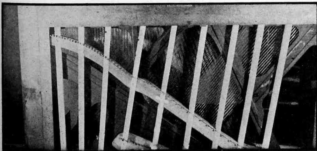
Fig. 6—The pick-up screws are all connected together with five mil diameter steel piano wire. The wire must not vibrate or rattle against the screws or supports if extraneous noises are to be avoided
