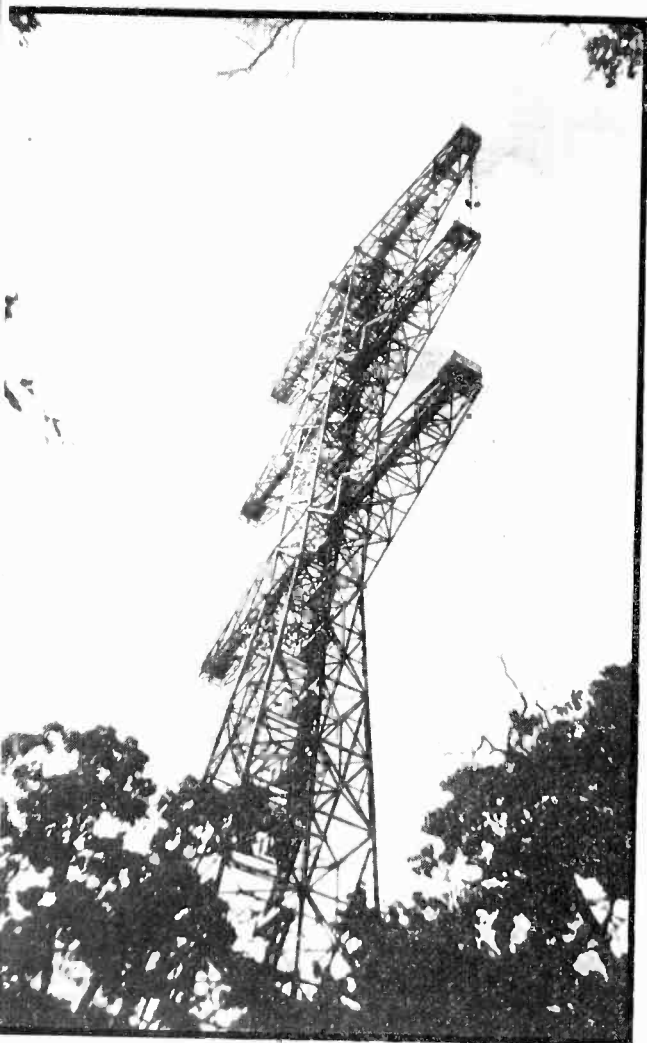
Four-hundred-foot steel tower atop Palisades supports turnstile antenna 900 feet above sea level. Radiating structure (see front cover) is supported between cross-arms at upper right
