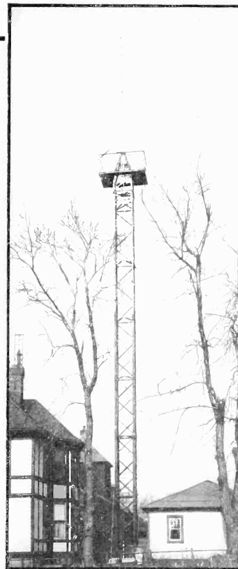
W2XCR, the 110-Mc 600-watt frequency modulation station of C. R. Runyon at Yonkers, which participated in the tests. The turnstile, above, is on a 100-foot mast
