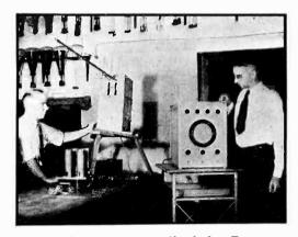
Members of the staff of the Engineeering Experiment Station at Purdue are developing ultrahigh frequency directional transmitters to be used for establishing landingbeams and markers for landing airplanes in fog
