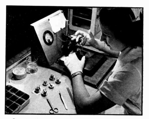
Focus of electron beams in X-ray tubes depends upon placement of filament in slot in focussing cup. In these Westinghouse units the accuracy of measurement is one ten thousandth of an inch
