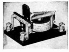
For Your Power Tubes. These light duty overload trip relays have a wide field of use as safety devices on electronic apparatus. Operation is unusually dependable. Scores of nationally known concerns rely on Leach Relays for protection.
